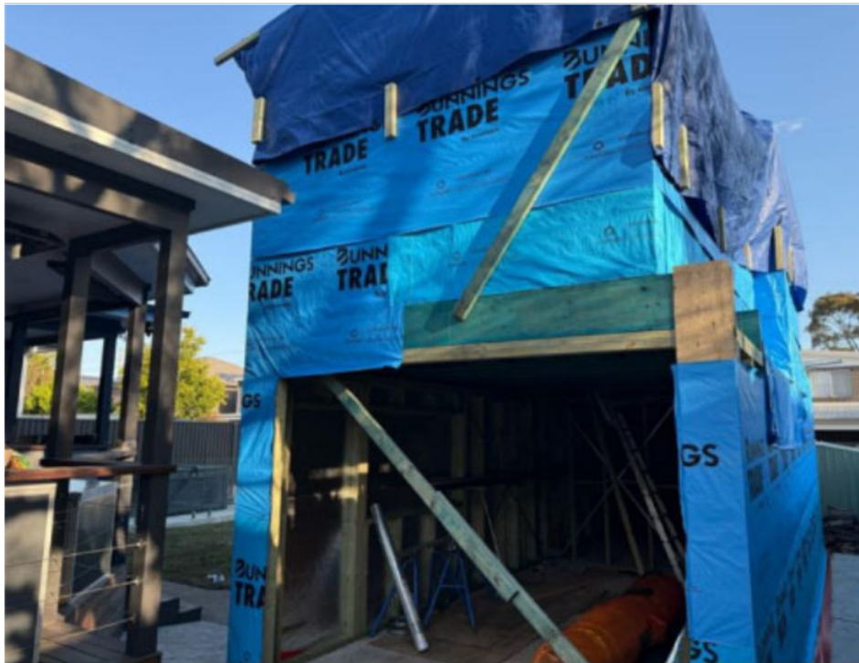
Figure 2: Existing structure at rear of site Source: Rockeman Town Planning
