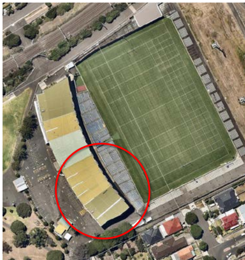
Figure 1: Area to be upgraded as part of Belmore Oval Sports Precinct Project
